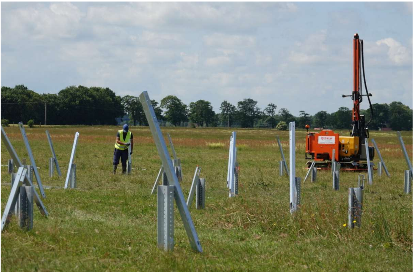
Plate 6: Example of a piling rig and piles
